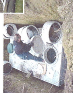
Replacing a septic tank and drain field
